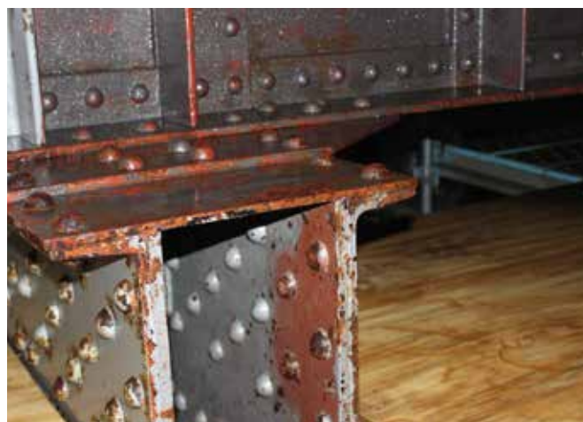
Box gantry rail bolt corrosion
