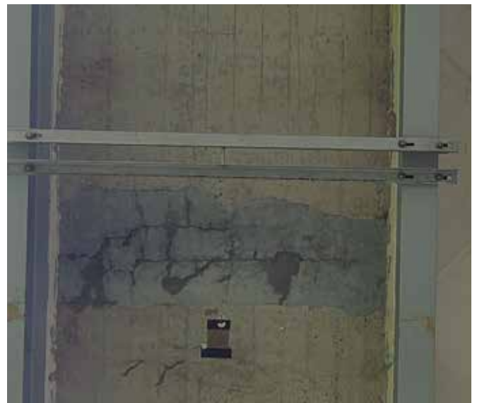
Water damage and concrete deterioration
