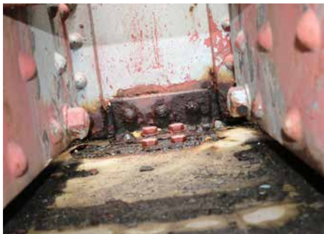
Box gantry rail bolt corrosion
