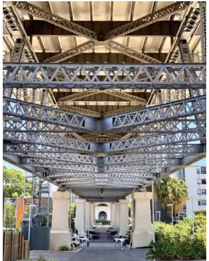
Steel frame of the Story Bridge
