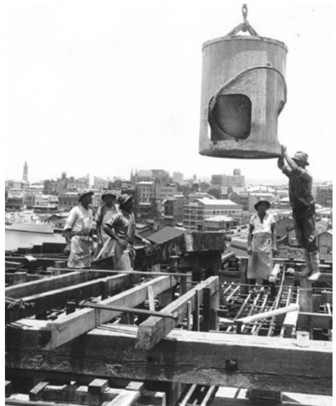
Concreting works on the Story Bridge – 1936
